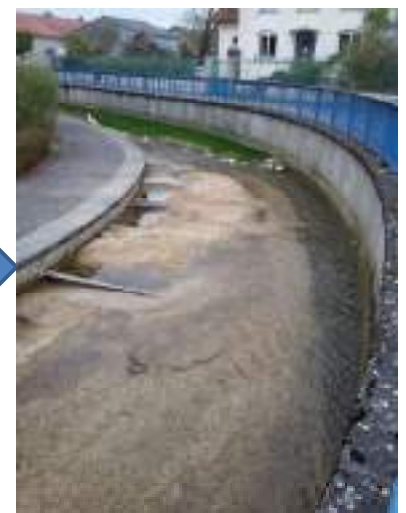
Picture 3: Groyne system in Fresnes-en-Woëvre (April 2017)
