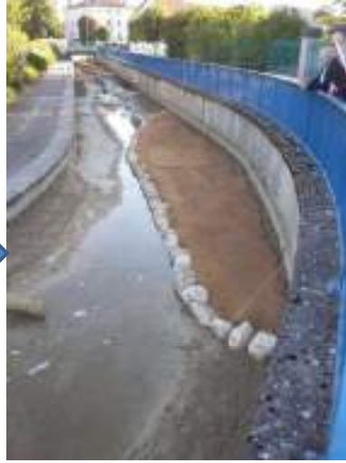
Picture 5: Riverbank filled with earth, covered with a geotextile membrane, girdled with stones in Fresnes-en-Woëvre (Sept. 2016)
