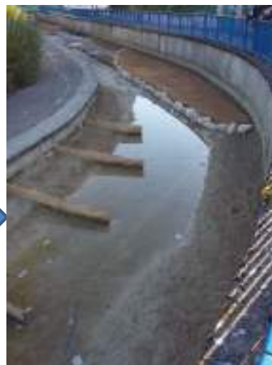
Picture 2: Groyne System in Fresnes-en-Woëvre (January 2017)
