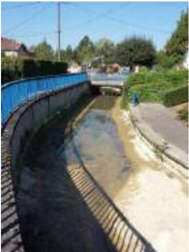
Picture 1: Fresnes-en-Woëvre before restoration (September 2016)
