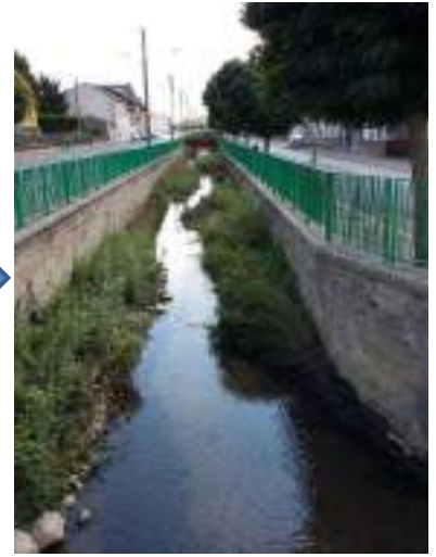
Stones and gravels riverbanks in Fresnes-en-Woëvre (September 2017)
