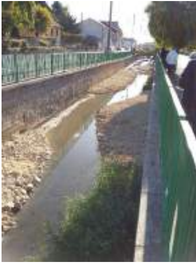
Stones and gravels riverbanks in Fresnes-en-Woëvre (September 2016)
