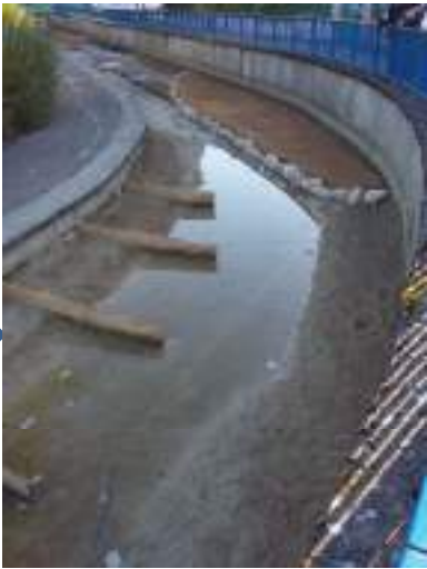
Picture 2: Groin System in Fresnes-en-Woëvre (January 2017)
