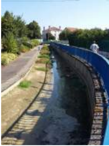
Picture 4: Fresnes-en-Woëvre before restoration (September 2016)
